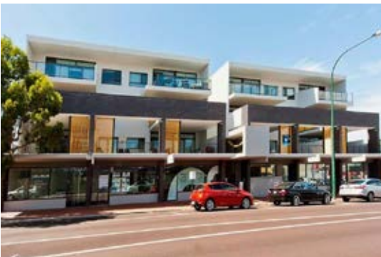
Image: Building height provisions in the PSP will achieve specific interface outcomes where appropriate.
