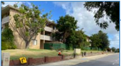
Existing higher density residential along Stirling Road.
