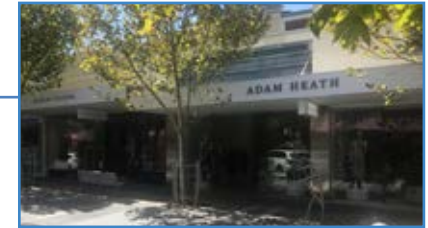
Existing character retail within the Bay View Terrace mall area.
