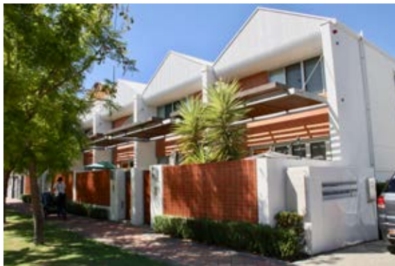
Image: Residential townhouses oriented to street
