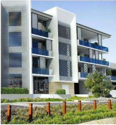
A combination of open, solid and adjustable elements facilitate optimised airflow.
